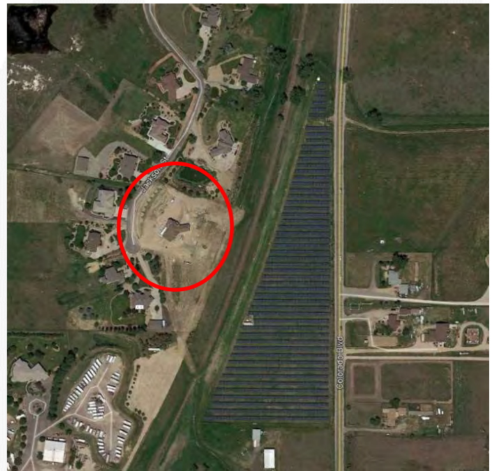
Brighton PV Solar, Adams County, CO June 2017
